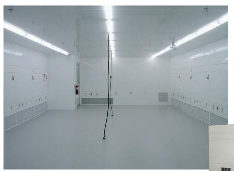
Low profile tunnel section with blowers in sidewalls. Combine multiple sections and end walls to form a cleanroom.
