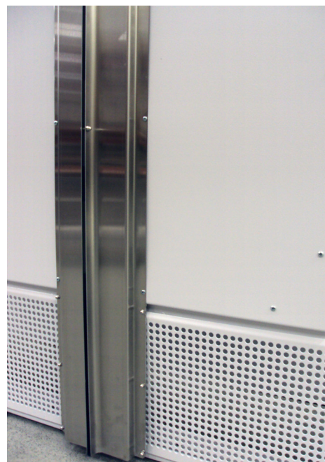
Figure 3 - Air shower vertical slot blower
