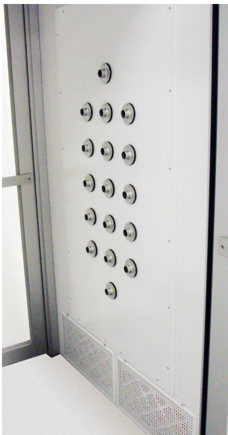
Figure 1 - Air shower side wall
