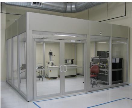
sophisticated modular room can be constructed in a week or two. Onsite assembly of a modular cleanroom is also less disruptive to surrounding operations in comparison to their fixed-wall counterparts.
